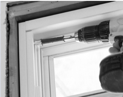
Block frame window installation: Block-frame windows don't have a fin. Installers use plates or screws to fasten the window to its opening.
